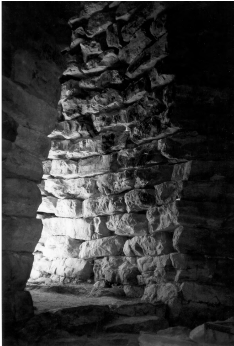
The central chamber of the nuraghe Is Paras, near Isili. In Santu Antine near Torralba, three such chambers are constructed at different levels, one above the other, an extraordinary achievement in dry-stone construction.
